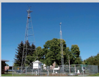
Meteorological observing station
