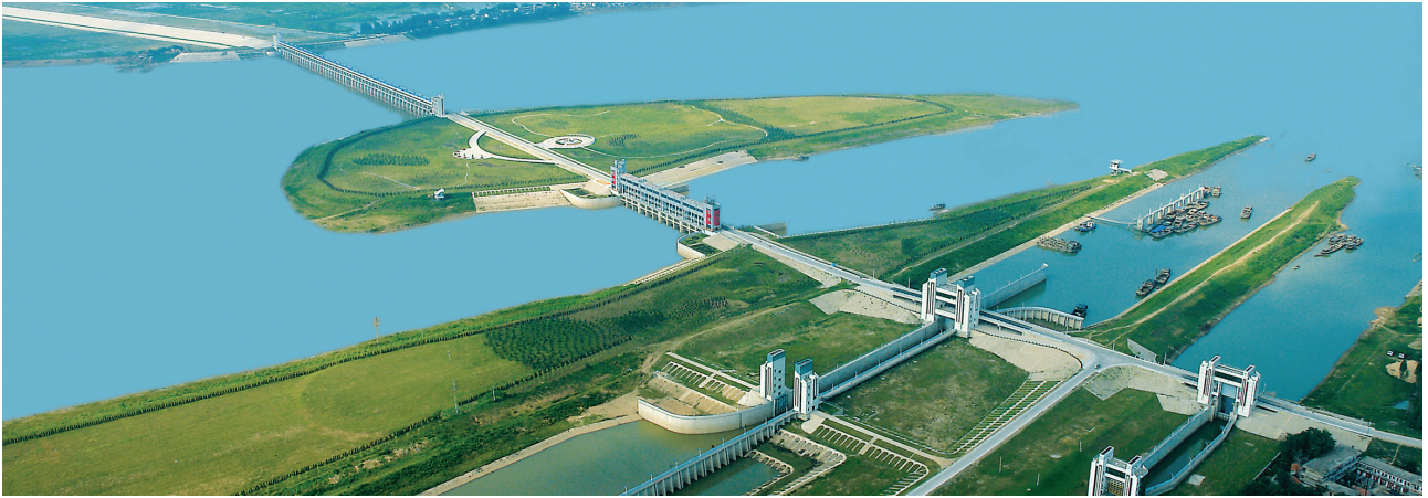
Linhuaigang Flood Control Works in Anhui Province
